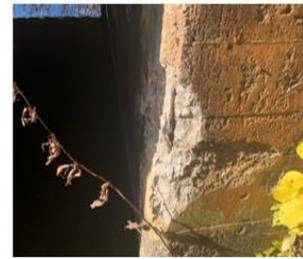
Photo 4: North East Abutment Wall Spalling
